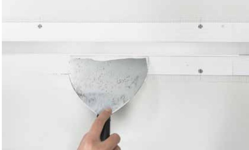
Step 4: Spackle, sand and Paint around the soft strip channel
